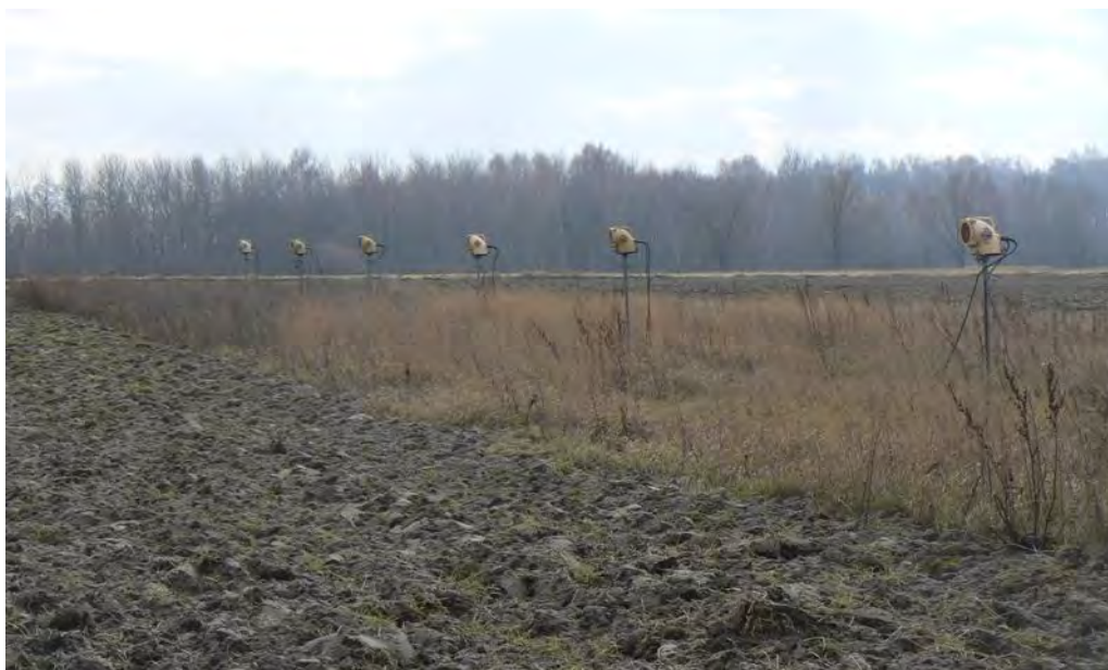
Photo 22. Construction of elements and the environs of ŁUCZ-2MU lighting system at the military aerodrome
