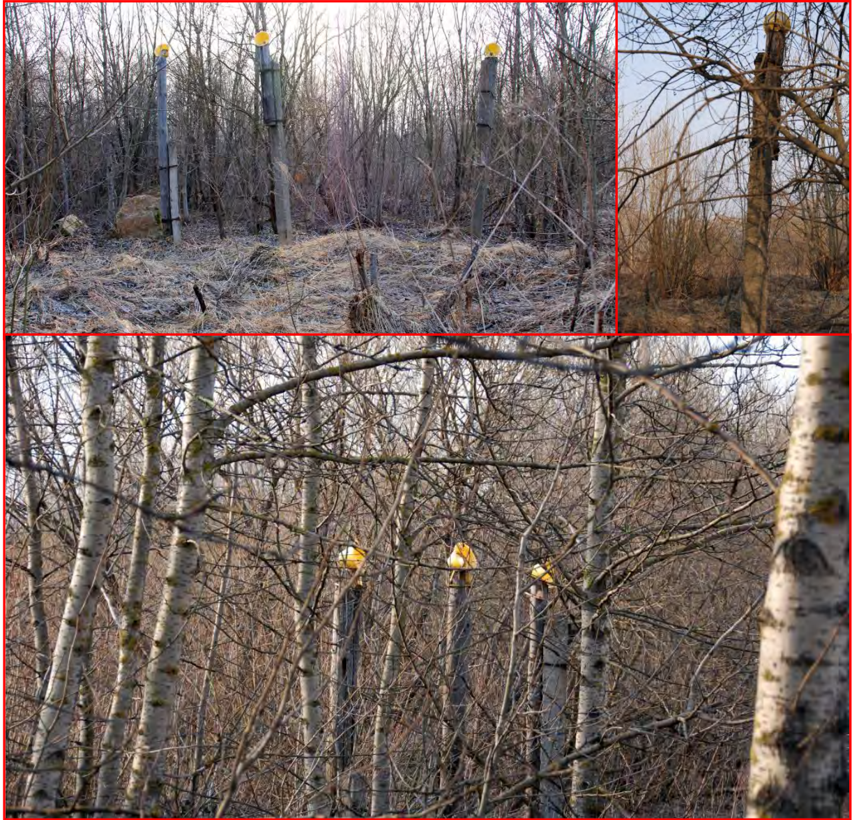
Photo 20. Navigation lamps obscured by trees and shrubs
