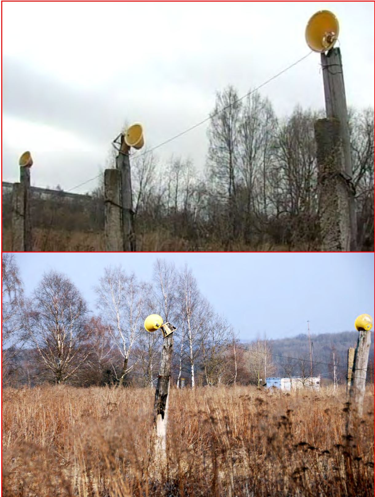
Photo 21. The technical state of approach lamps
