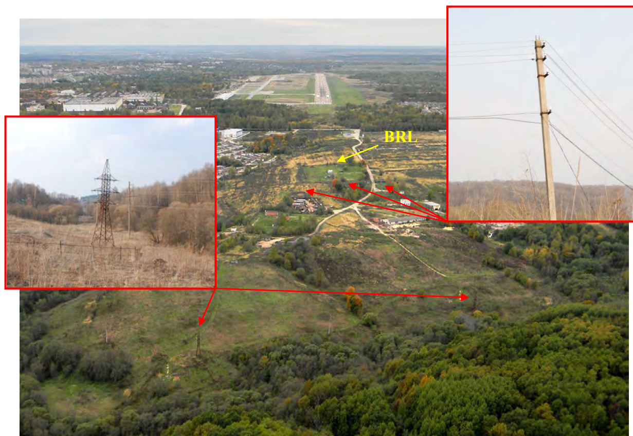
Photo 17. Location of power lines and low-voltage lines relative to Inner NDB
