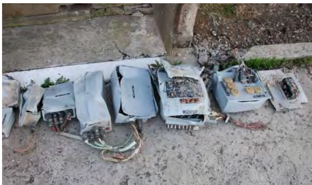
Fig. 30. The control boxes of the electrical system
